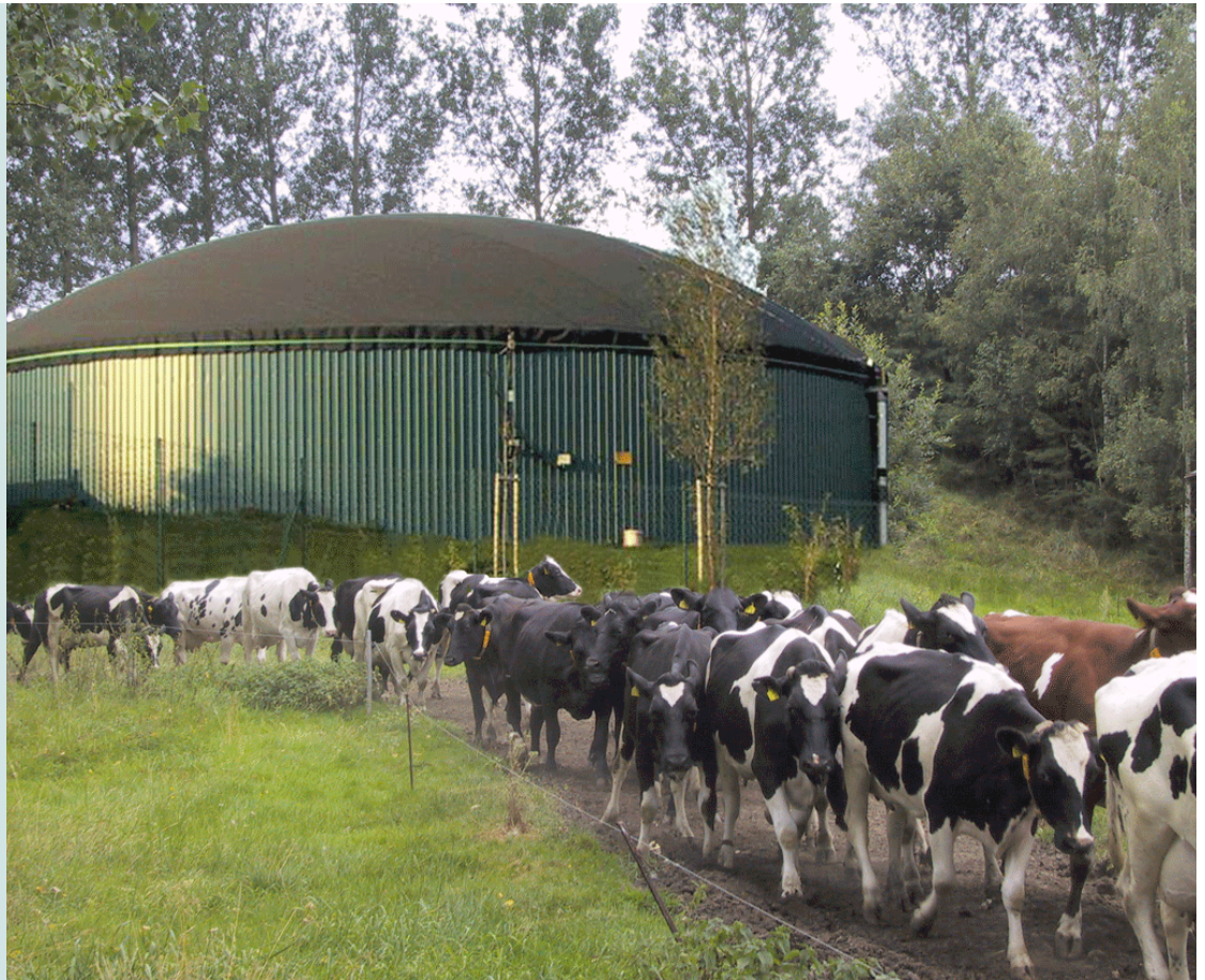
Anaerobic digester (ADG) plant producing biogas from animal waste
